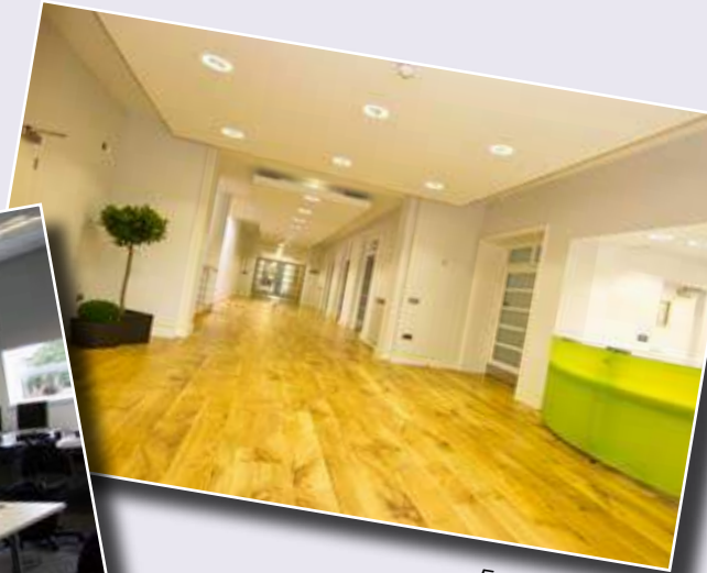
Entrance Hall (After)
