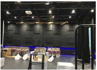
In the drama classroom existing recessed light fitting were replaced with dimmable LED panels and mirror lights in the form of LED strips. Again the lighting was controlled via wall mounted scene set plates to enable different scenes to be selected.
